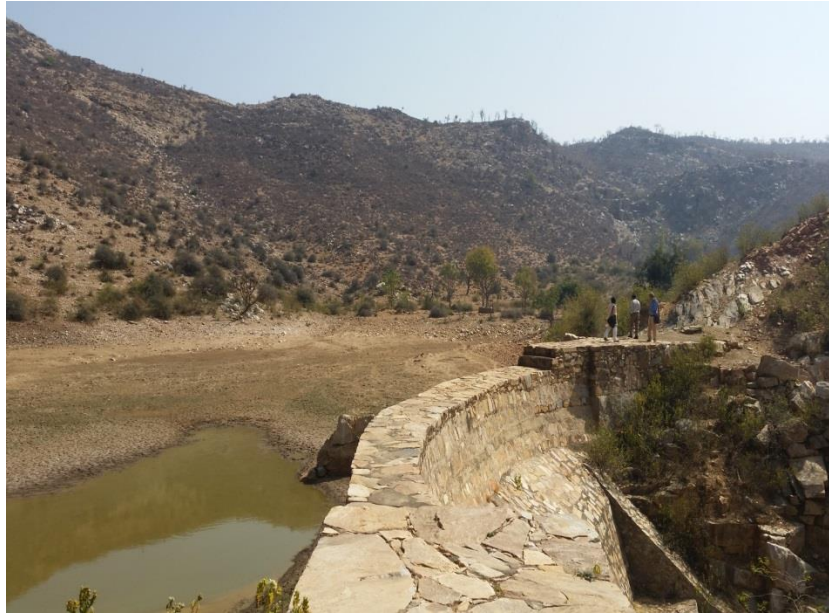
Figure 21. Cement Reinforced Earthen Dam in Bhauta
