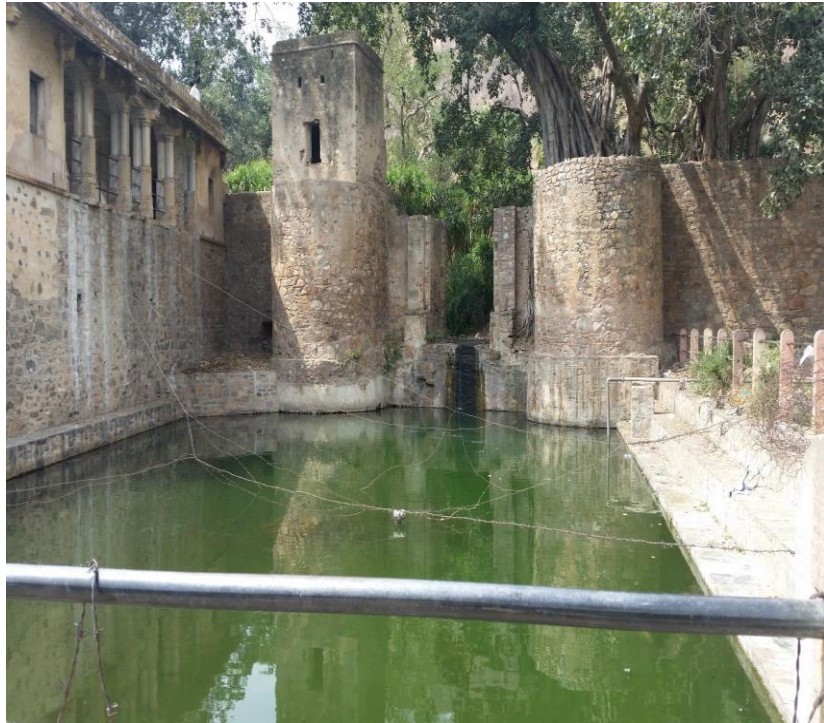
Figure 18. Catchment Dam in Bhangard
