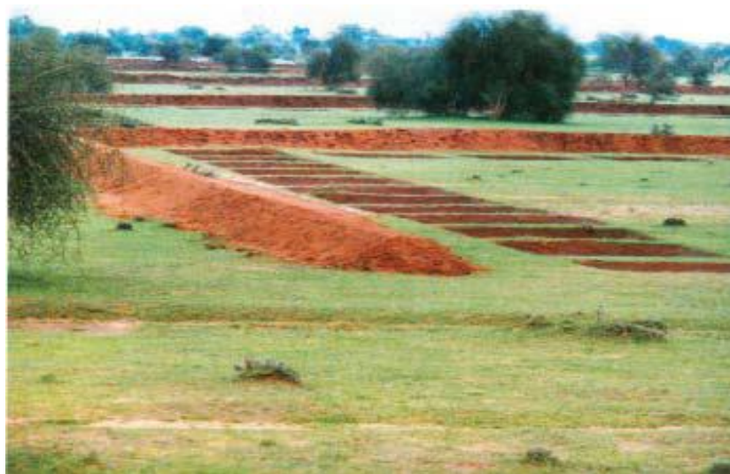
Figure 8. Newly Constructed Chauka System
