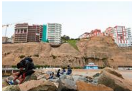
Figure 5. Illegal real estate development on the cliffs of the district of Barranco
