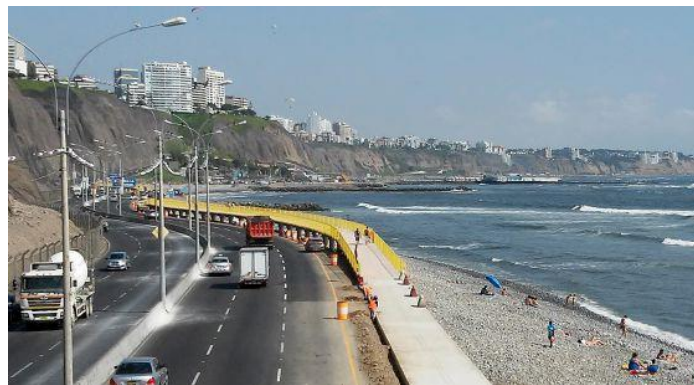
Figure 7. Sports facilities built by the Metropolitan Municipality of Lima in 2015, obstructing the view of the seaside (Source: Diario El País , 2015)
