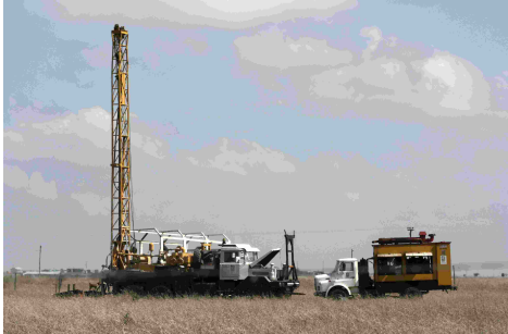
Drilling another borehole
