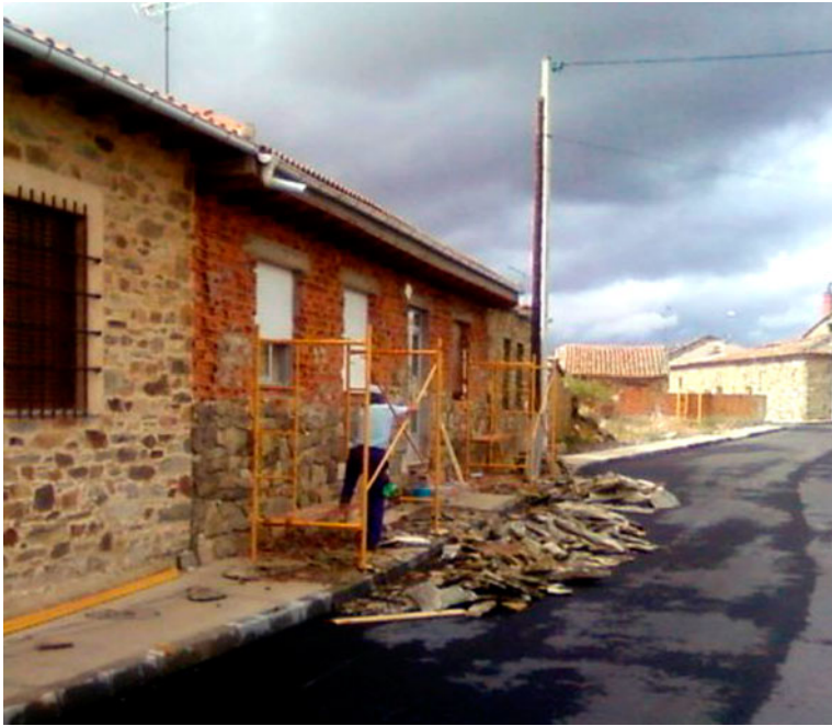
FIGURE 7 A man gets rid of the stone coverage of his modern house, leaving the ‘ugly’ bricks and concrete in sight.
