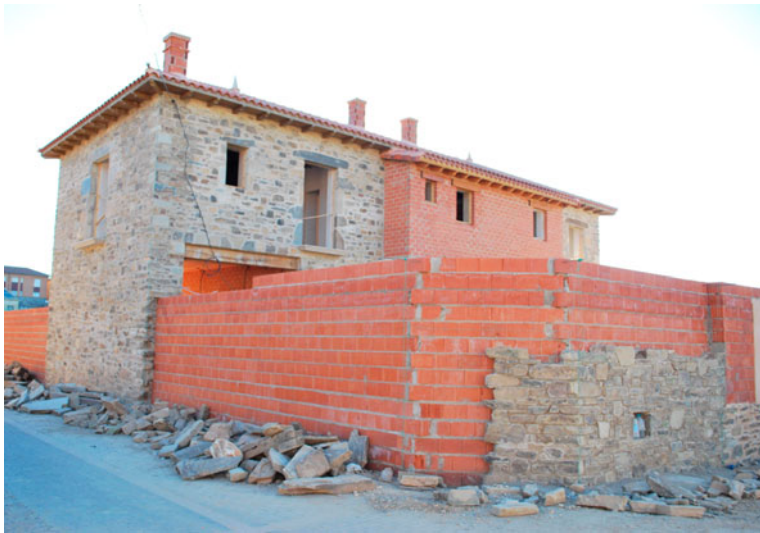
FIGURE 6 Postmodern house built with a modern structure and covered by a traditional-looking envelope of vernacular tiles and stones.
