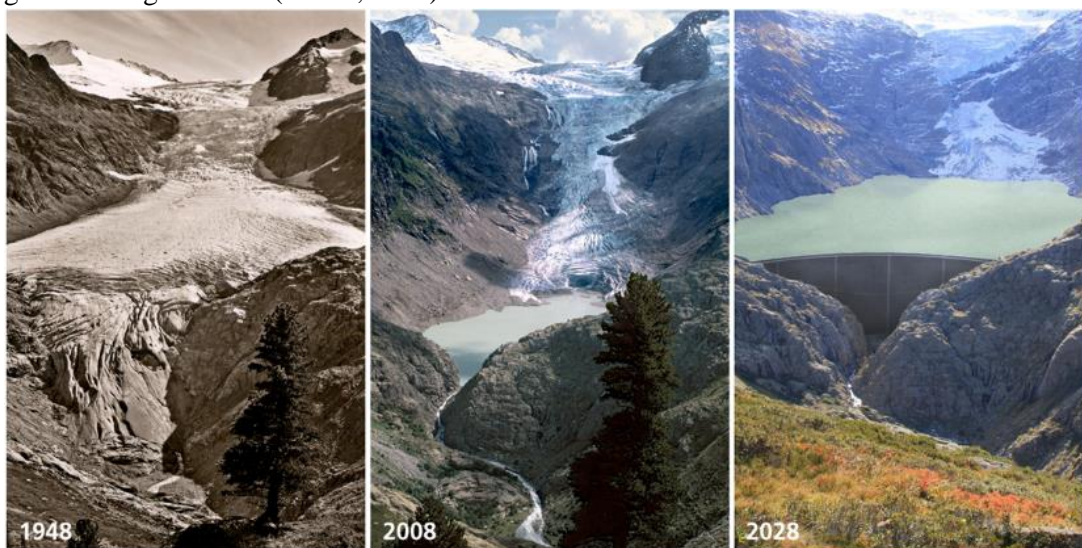
Figure 1: Planned hydropower dam at the Trift glacier in Swiss Alps, with the glacier in 1948 (left), lake in the glacier forefield in 2008 (middle) and with proposed full reservoir (right). (Source: Kraftwerke Oberhasli AG).
