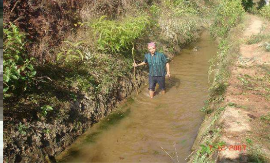
Photo 2: Canal Cross section
