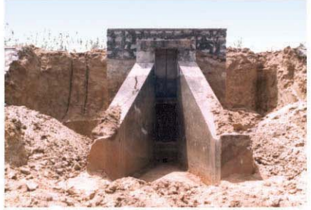
Damaged sluice
