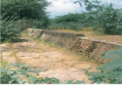
Damaged weir
