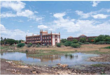
Encroachments by Government buildings
