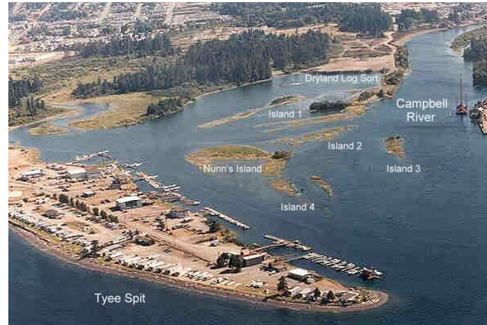
Fig. 1. Aerial photo of the Campbell River estuary looking south. Shown are the constructed islands in relation to Tyee Spit, Nunn's Island, and the dry land log-sort area (6 August 1998).
