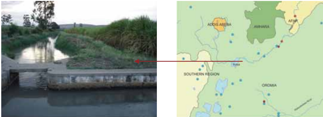
Figure 21. Wonji Irrigation Scheme.
