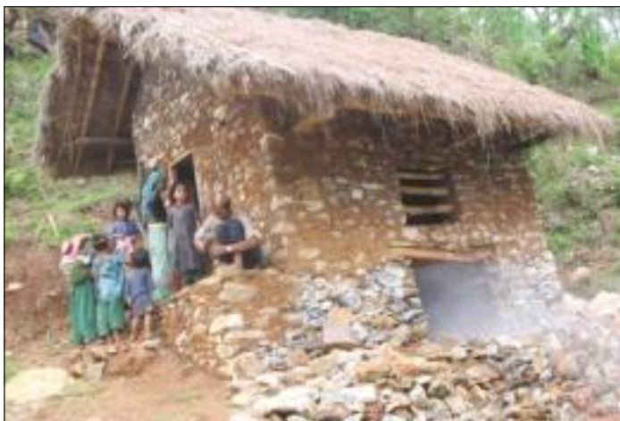
Pani Ghatta (Water Mill) construction support at Korhabang, Rolpa district
