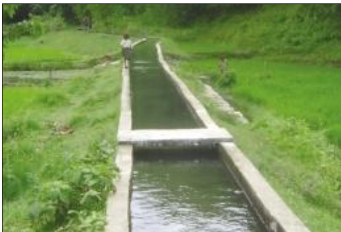
Irrigation canal built in Bayarban, Morang district
