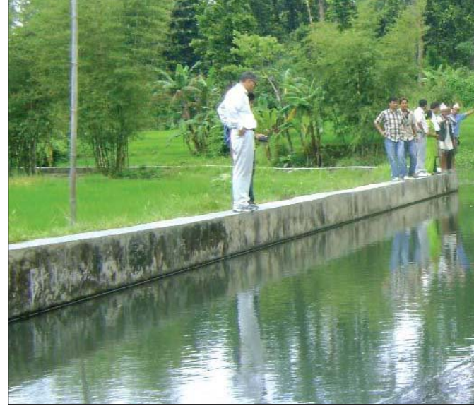
Participatory monitoring of the canal operation
