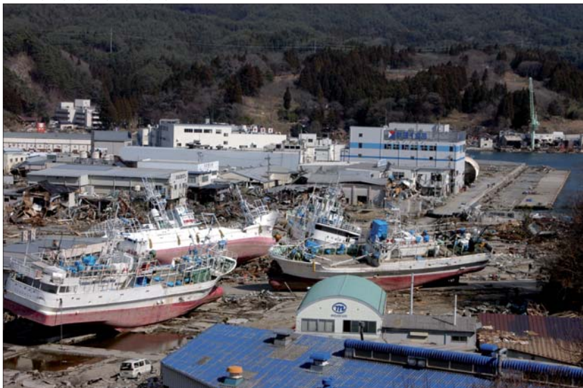
Fishing vessels thrown off the Kesennuma port, Japan. The road to the commercial wharf was made impassable as the ground near the fish market sank about 1 m
