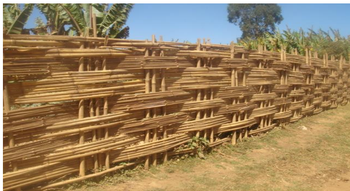
Figure 4 The type of fence constructed from bamboo
