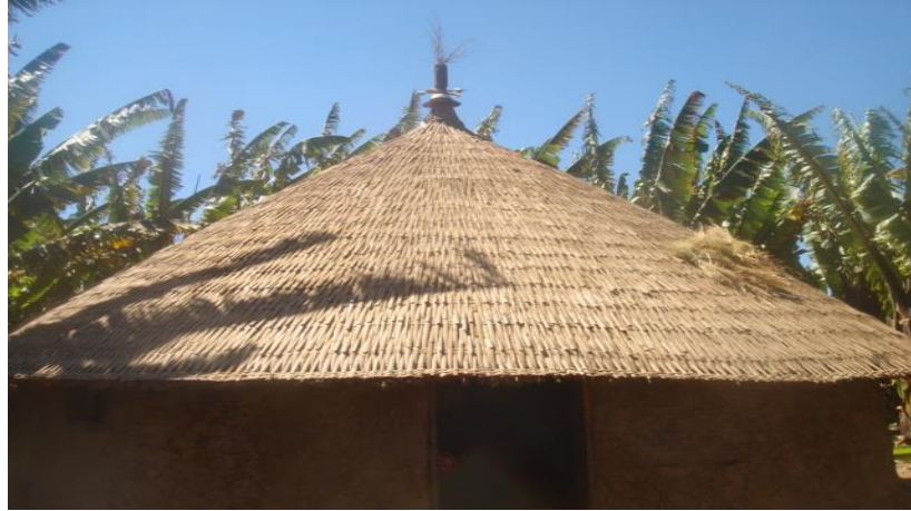
Figure 3 Traditional house constructed from bamboo and other material
