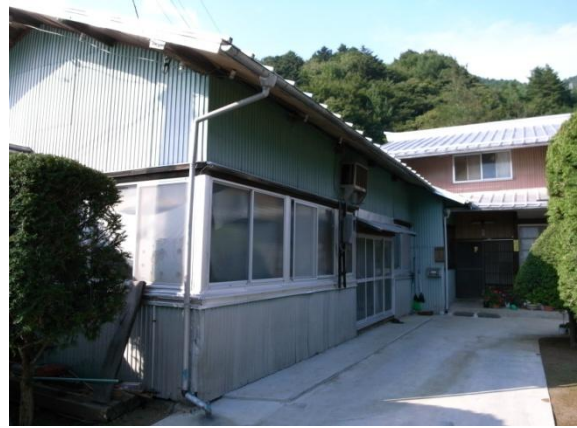
Fig. 5. A factory connected with its owner's residence.
