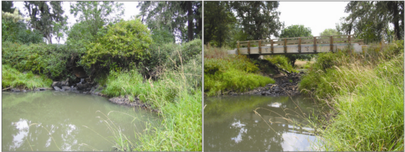
(a) Culvert (before)
