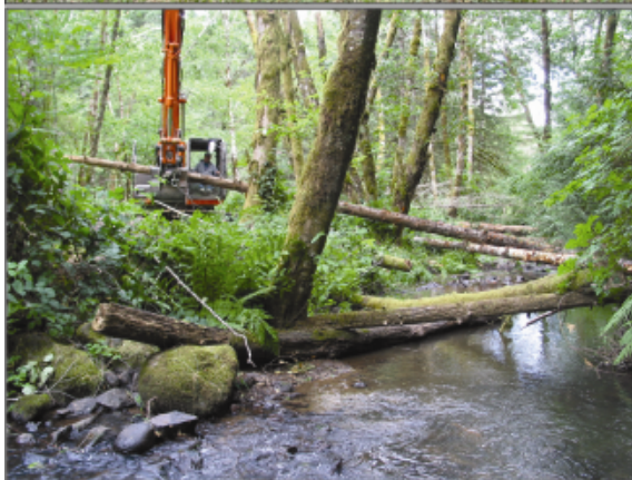
(c) Large wood placement for fish habitat
