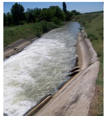
Fig. 4 – Secondary canal belonging to the Sayram-suvi WCA
