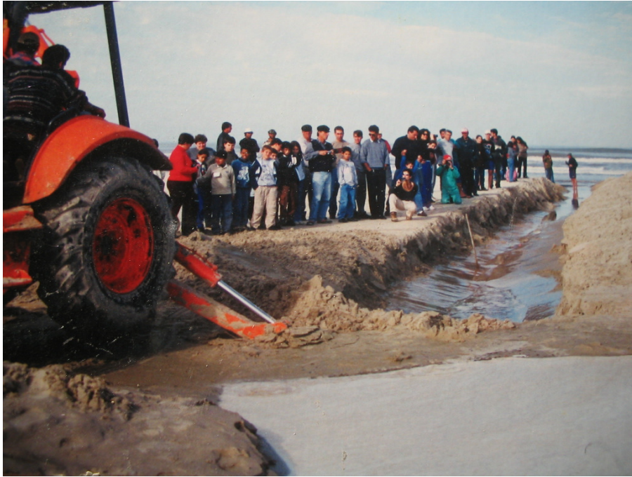
Figure 3: Backhoe opening a ditch to connect the lagoon to the sea
