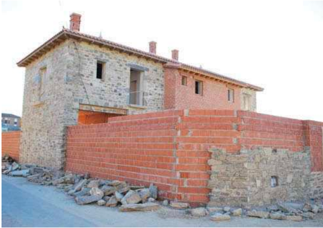
Figure 2. Supermodern house imitating maragato architecture built from scratch in Val de San Lorenzo. The design and materials are modern, but its external appearance is intended to look vernacular. Source: Author.
