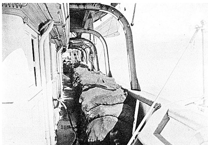
Figure 2.—Coal sacks were stacked in the gangways on the deck of the Albatross in 1914. E. Lester Jones wrote "...the Albatross is a coal burner [which] makes her expensive to operate and lessens her efficiency, particularly on account of a reduced steaming radius." (Jones, 1915).
