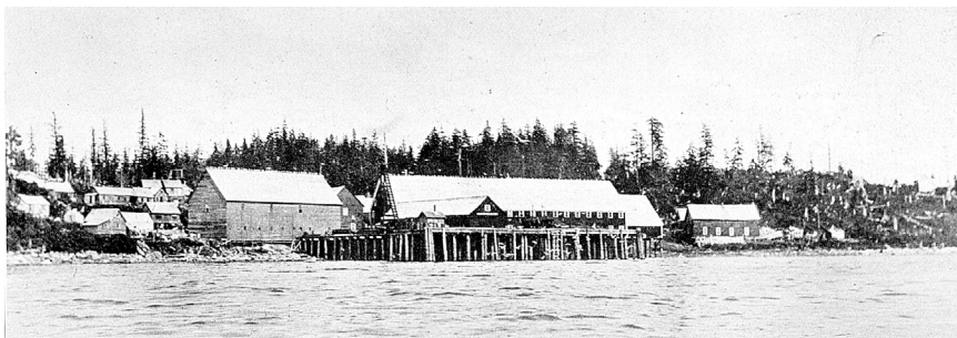
Figure 8.—This view of Yakutat’s cannery in 1914 is typical of the illustrations in the reports of Moser and Jones. Often these U.S. Fish Commission photographs are the only historical record of what these canneries looked like (Jones, 1915).
