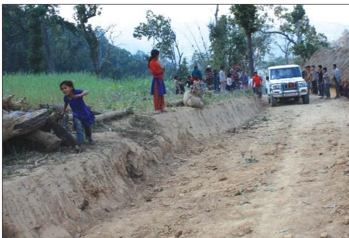
Newly constructed agriculture road under FASIRIN project in Kalidamar VDC, Surkhet
