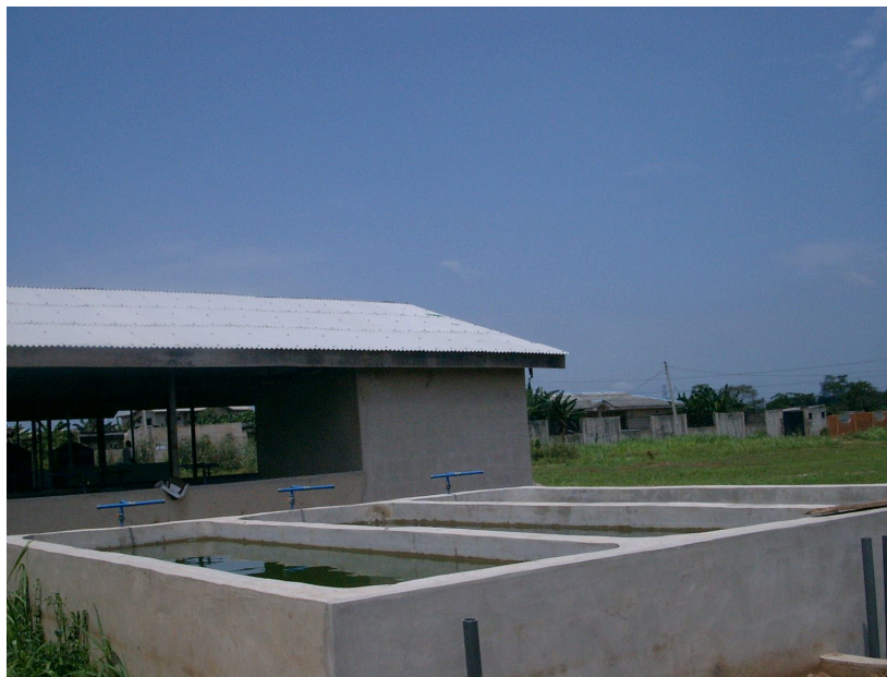
Fig. 3. A flow-through concrete tank for growing the African catfish, Clarias gariepinus .
