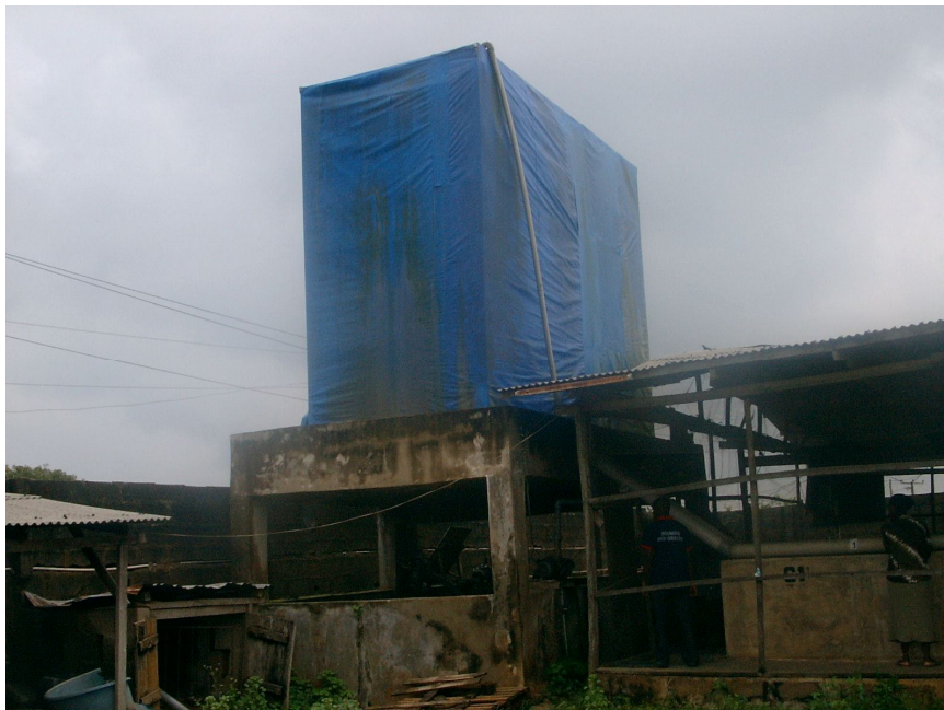
Fig. 4. External view of a Water Recirculation Aquaculture System (WRS) facility.
